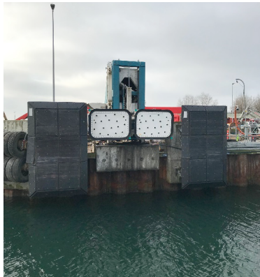
Figure 21a – Example of modern mooring. Ferry harbor Spodsbjerg, Denmark
