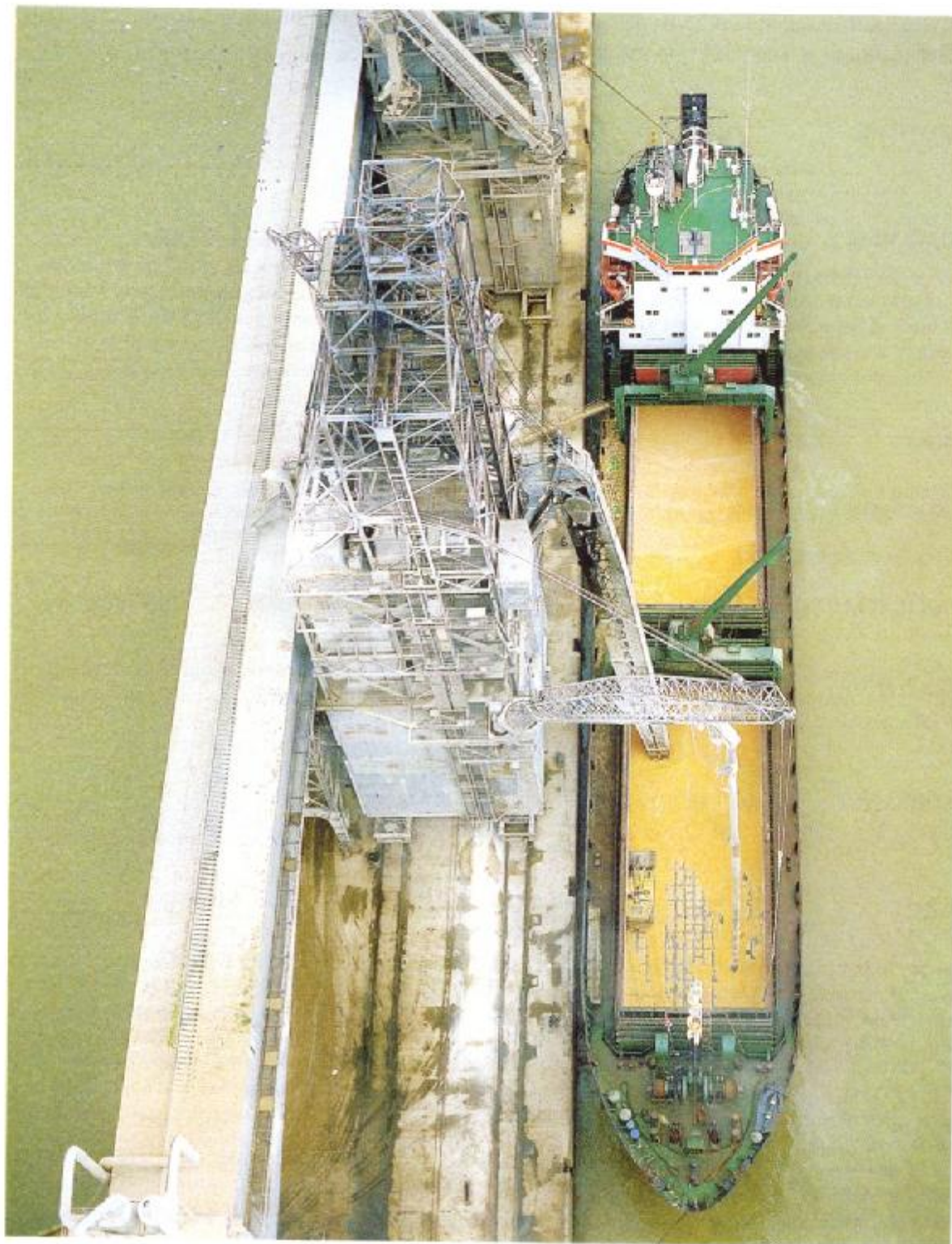
Nearing Completion of Automated Grain Discharge (Photo: Forth Ports Plc).
