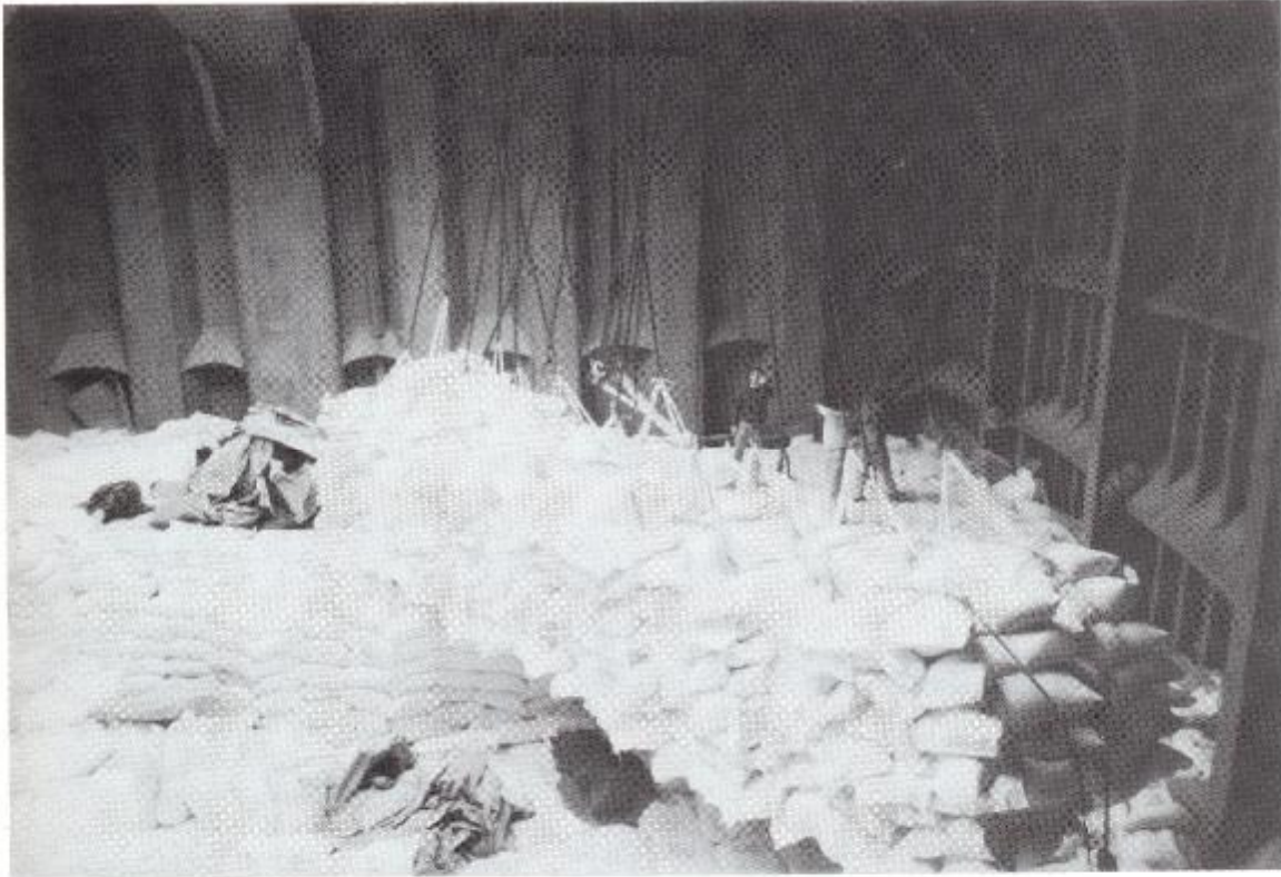
Multiple sling discharge.
