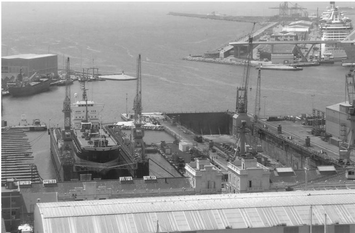
The vessel 'Carantec' lies in the floating dry dock in the Port of Barcelona, Spain. The empty graving dock lies to the right of the floating dock. The caisson is seen closed facing the harbour entrance.
